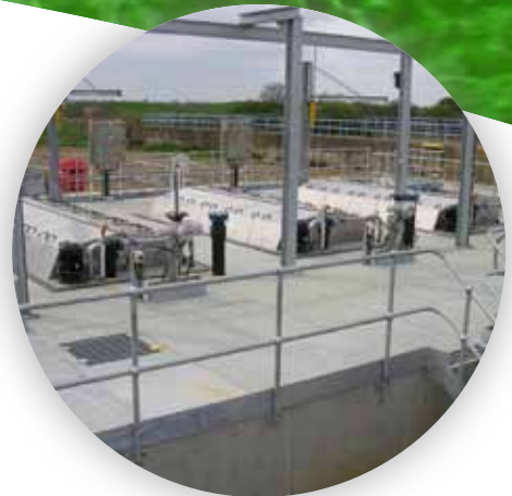
Hydretech Discfilter type HSF2212 for installation in a concrete basin.
