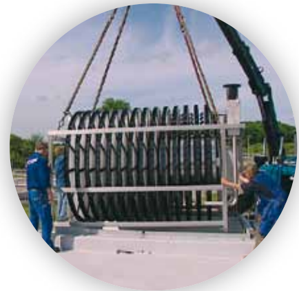
A HSF2214 being installed in small WWTP in Denmark.
